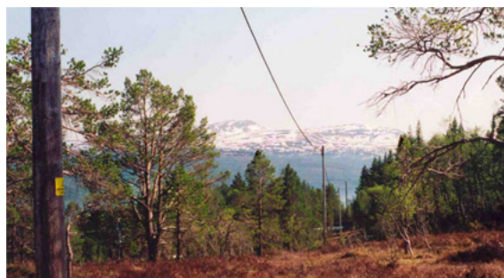
Fig. 11. Universal cable installation in remote area
